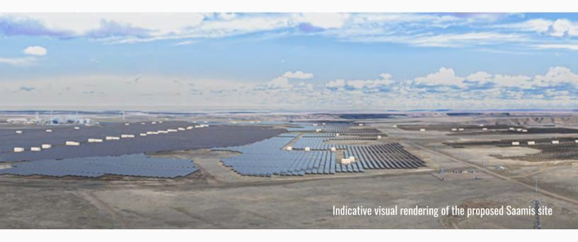
The Project will have a total generation capacity of approximately 325 MWac, comprised of solar PV modules installed in a mixture of fixed tilt and single axis tracker racking systems.
